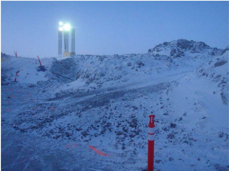
Photo 2: View of central access ramp into the North Dam key trench. Note that the base of the ramp will be required to be pulled back at a later date as it is within the core footprint. The base of the access ramp is construction with transition material (compaction is required on this ramp).
