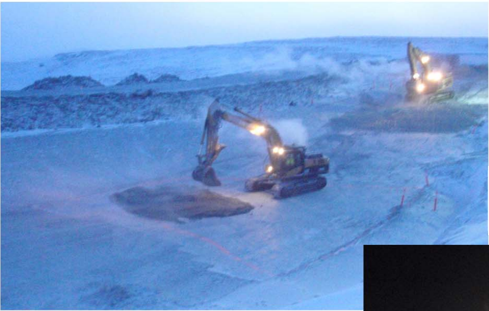
Photo 9 (above/ top center): Excavator spreading the first 2012 load of frozen core in the key trench, ~ SW view.
