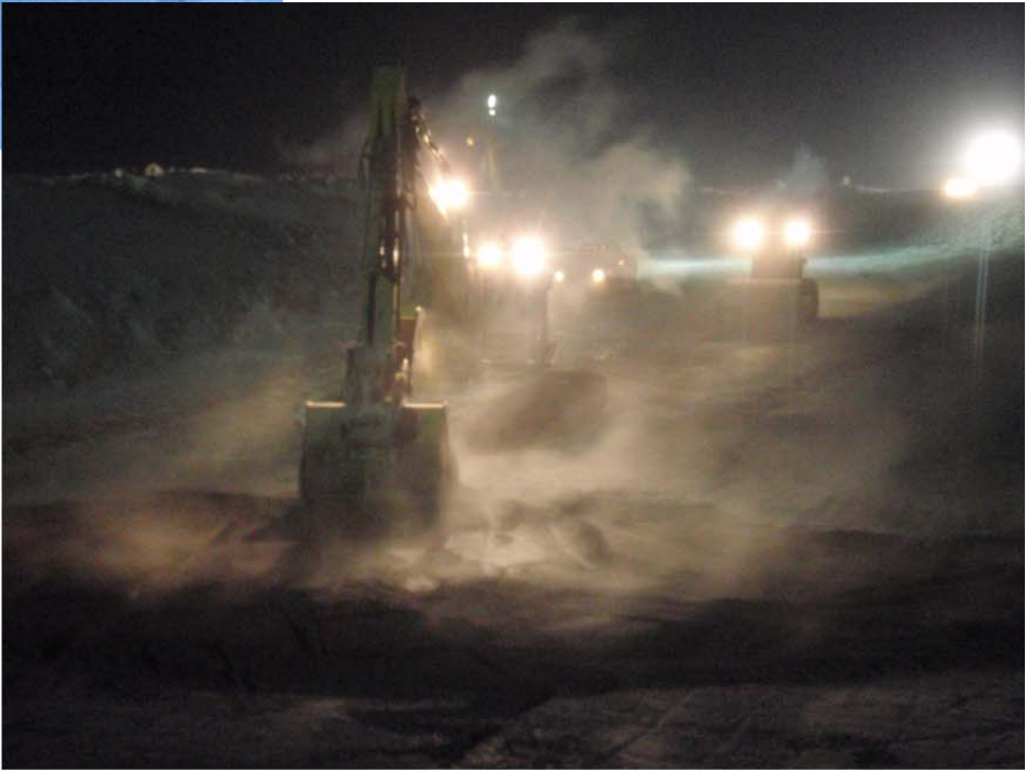
Photo 10 (below/ center right): Excavator working to place frozen core material (~3.5 loads) in the central area of the key trench; ~ NE view.
