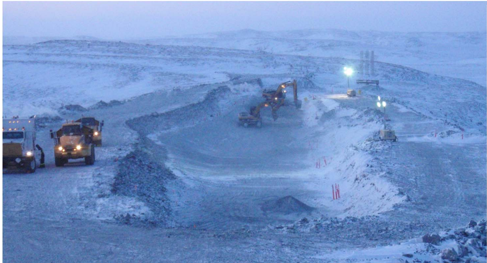
Photo 1: ~WSW view down key trench centerline. Note excavators in background removing/ scraping down 5/8" material.
