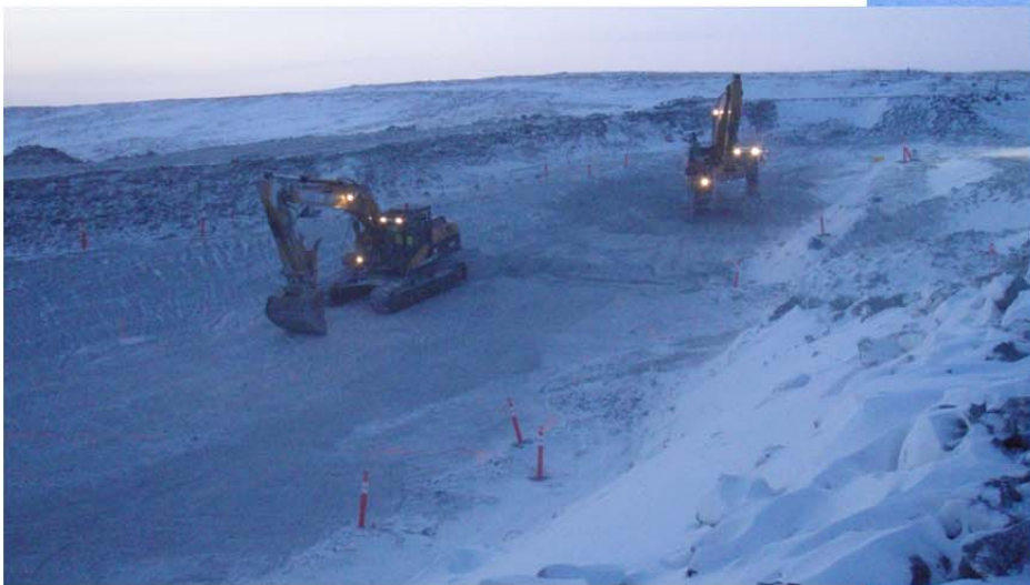
Photo 4: ~SW view of excavators scratching frozen 5/8" material from the key trench base. Note that the excavator in the forefront has a finishing bucket while the excavator in the back has a toothed bucket.
