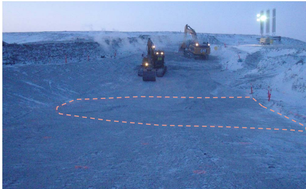
Photo 3: ~W view of cleaning activities around the central key trench area (i.e. WSW of station 0+85). Note that the area where placement occurred today is outlined by the light red dashed line.
